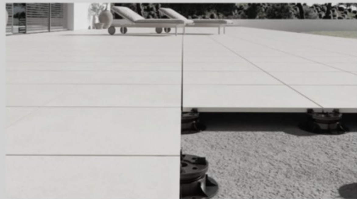
Designed a perfectly flat, free-draining pool terrace using a raised technical flooring system that elegantly conceals underlying slopes and utilities while ensuring easy maintenance access.
